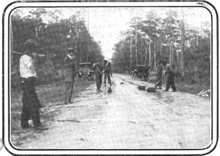
The oiling of the course is being carefully and evenly done
